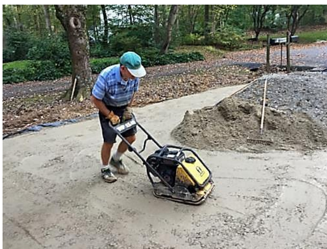
Ron Marlow compacting aggregate.
