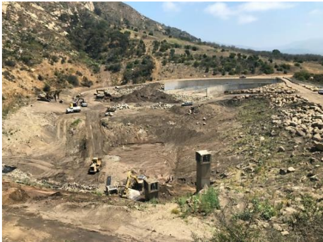
Santa Monica Debris Basin being maintained after debris flow (Final stages of Phase I Work)
