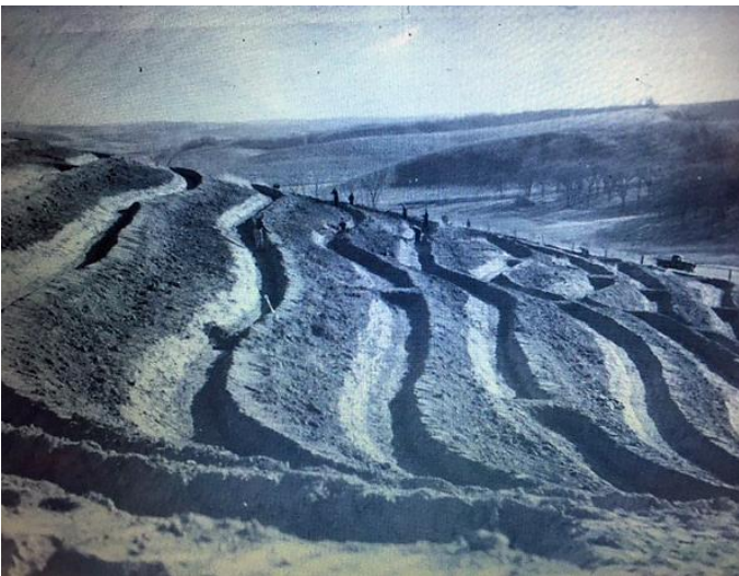
CCC Hand dug terraces on the Dale DuVal family farm.
