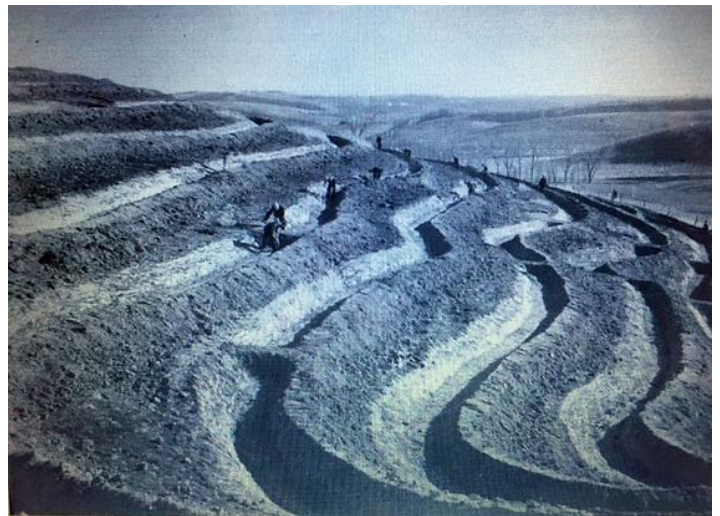
CCC Hand dug terraces on the Dale DuVal family farm.
