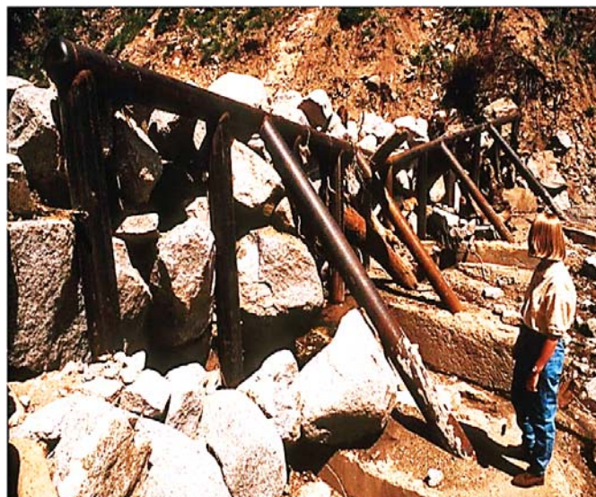
After: Trash rack full of boulders after storm event
