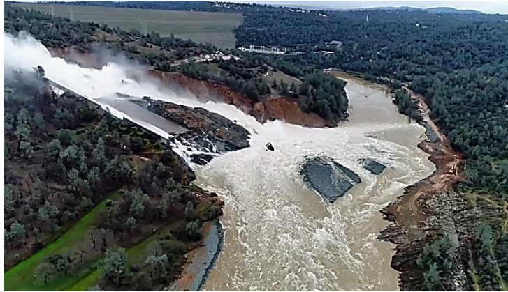
"Debris Pile" blocking channel at base of Primary Spillway.
