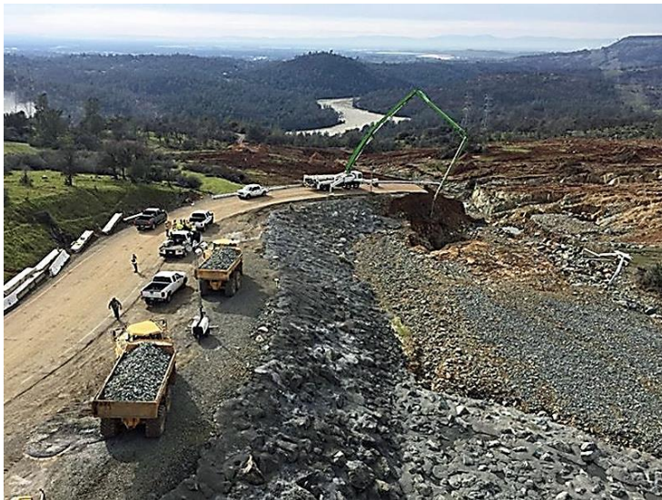
Repair work being done on eroded areas below Emergency Spillway.
