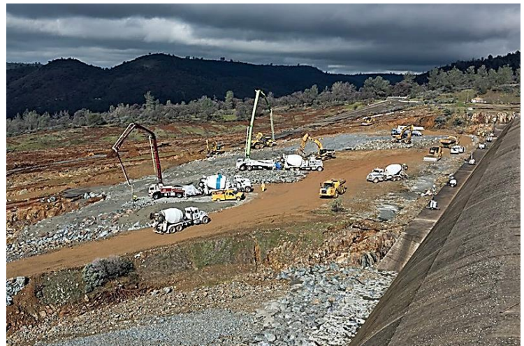
Repair work being done on eroded areas below Emergency Spillway.
