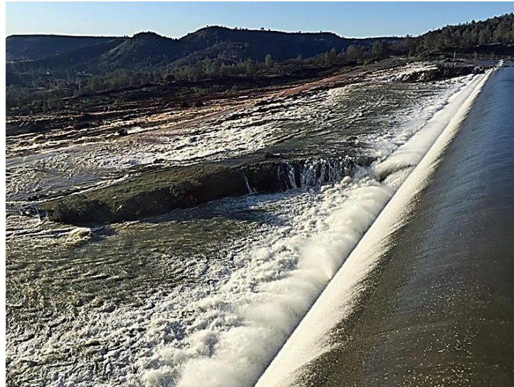
Peak flow over Emergency Spillway, approx. 10,000 cfs.
