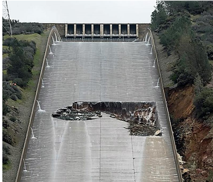
Primary Spillway Damage
