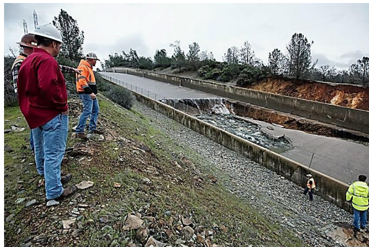
Primary Spillway Damage
