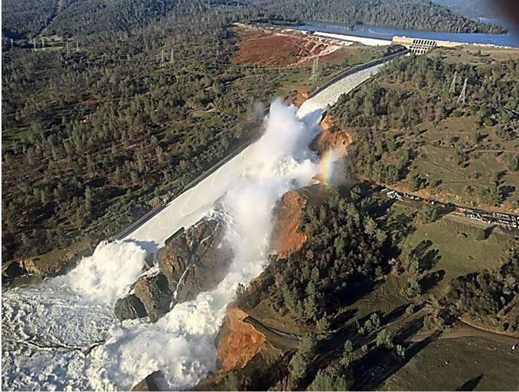
The damaged primary spillway at 100,000 cfs after evacuation orders!
