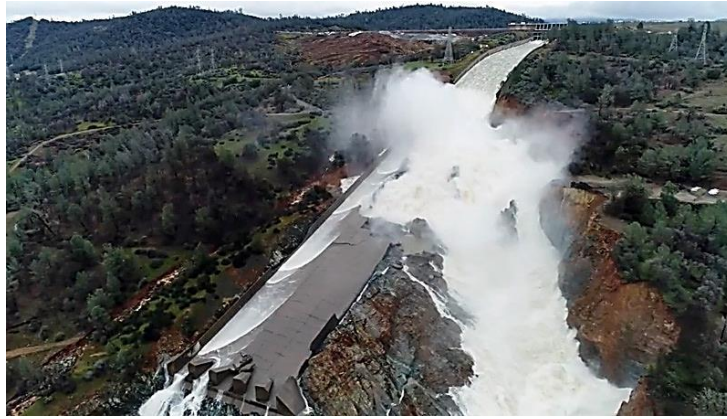
Primary Spillway after eight days at 100,000 cfs, now discharging at less than 100,000.cfs.
