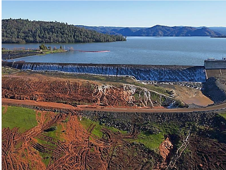
Early stages of flow over Emergency Spillway.
