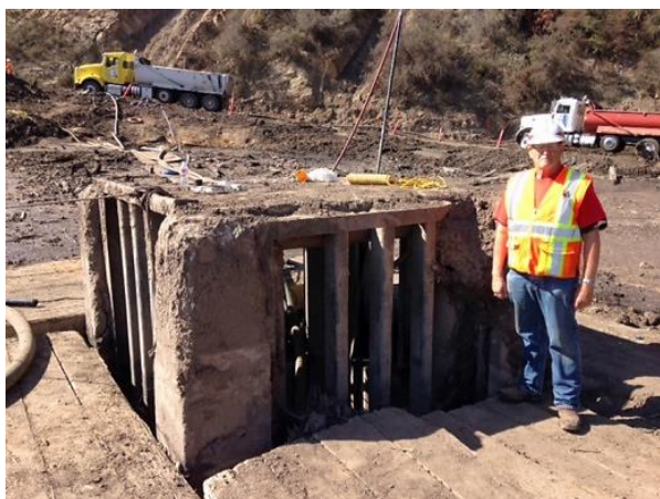
Main principal spillway tower, major blockage
