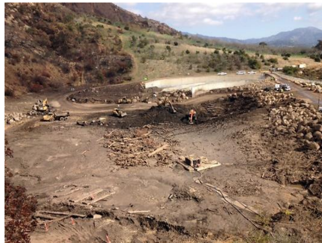
Overview of Santa Monica Debris Basin restoration work on February 18, 2018. Note the exposed top of the principal spillway tower near the center of the photo
