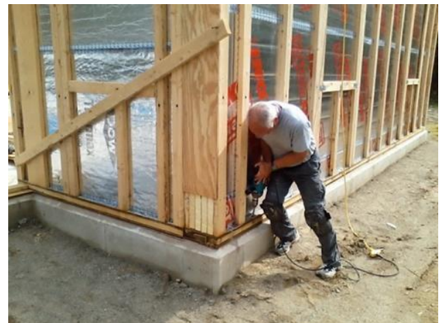
A sample cross-section of exterior wall of Art Taylor's house. The 8 inches of styrofoam sandwiched between two layers of 2x4s and the inside sheetrock and outside siding bring the R value of the walls to well over 50.
